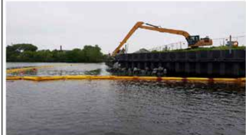
Photo 4: R6 material placement via long-reach excavator, facing west.
