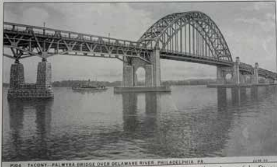
It was not until this structure was complete that the areas west and northwest of the Disston Estate became ripe for settlement. The community was no longer viewed as a suburb. Along with the Roosevelt Boulevard extension and creation of the Market-Frankford elevated line, the new bridge made access convenient from all points. The Tacony-Palmyra Bridge opened during a torrential rainstorm on August 14, 1929, with a gala ceremony, which included dignitaries and citizens.
